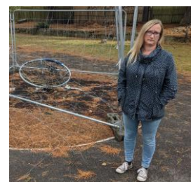
Unrepaired arson at Moordown Rec: Kate Salmon is asking the Council what's to be done
