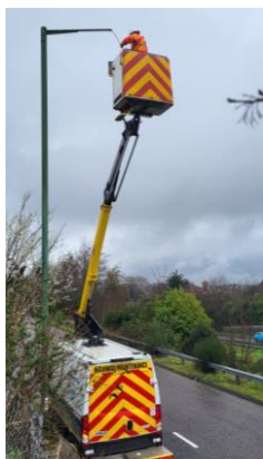
Streetlights being renewed and fixed along Wessex Way
