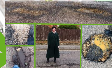
Kate has reported potholes and road defects across the ward: Wimborne Road, Castle Road, Gresham Road and Malvern Road
